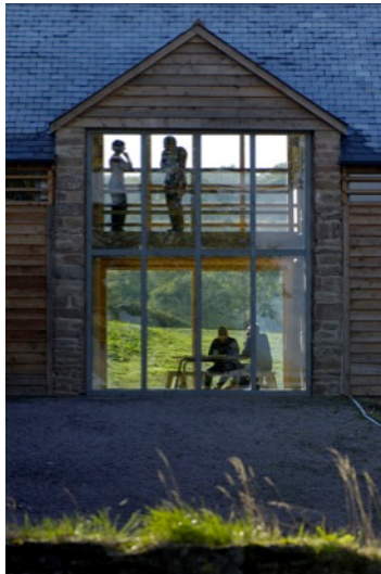
West Office - Barn Ecological refurb
